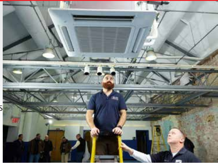
Ceiling cassettes were used throughout the Bronx Neighborhood Government building. This is in the Carriage House.
