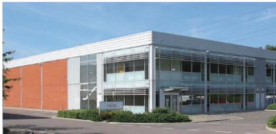
Building where FGAC(UK) resides
