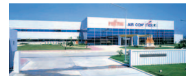
Fujitsu General (Thailand) Co., Ltd. Fujitsu General Engineering (Thailand) Co., Ltd.
